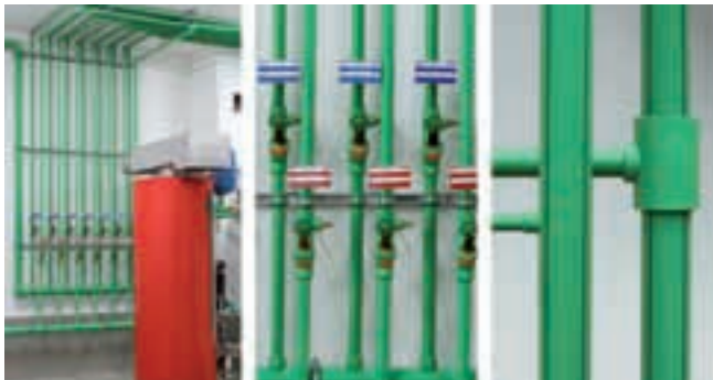
...to risers, installed with fusiotherm®-composite pipe, with conventional high rise or high rise carried out with the fusiotherm®-manifold system...
