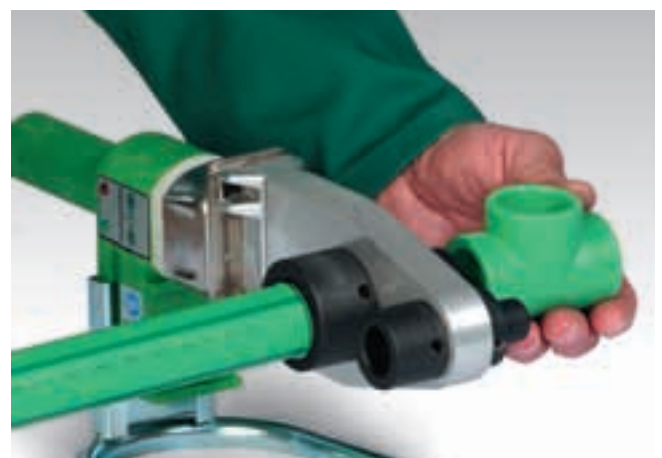
Heating-up of pipe and fitting
