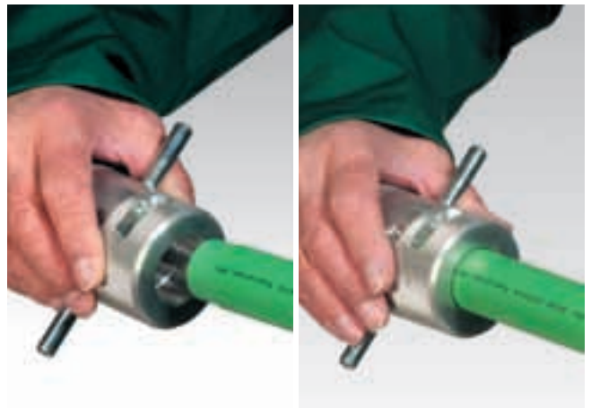
Peeling of the aluminium-PP-composite-layer (Necessary only for stabi-composite pipes!)
