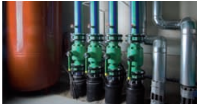
Flange connections and transition joints enable the connection of all components to the central heating system and on the floor.
