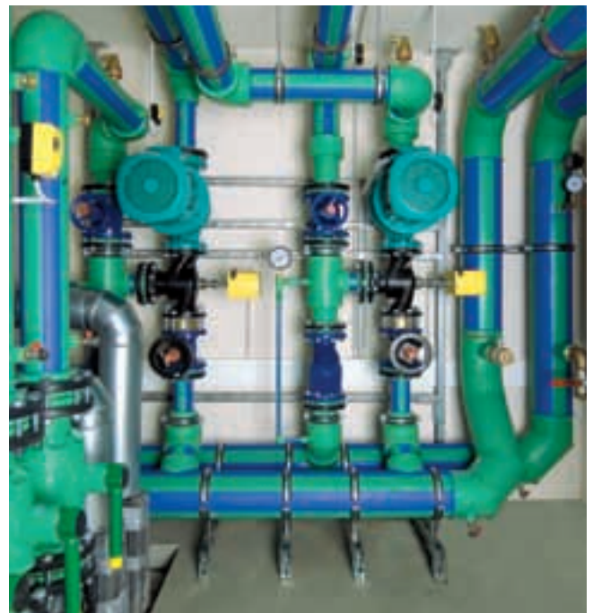
Manifold construction with fusiotherm®- and climatherm-faser composite pipe and big ball valve
