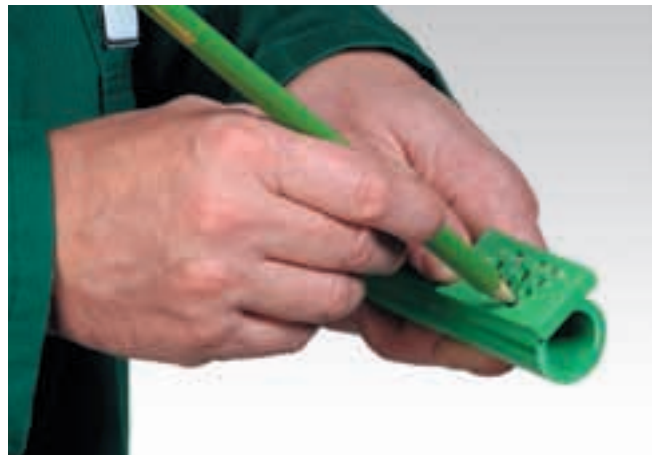
Marking of the welding depth
