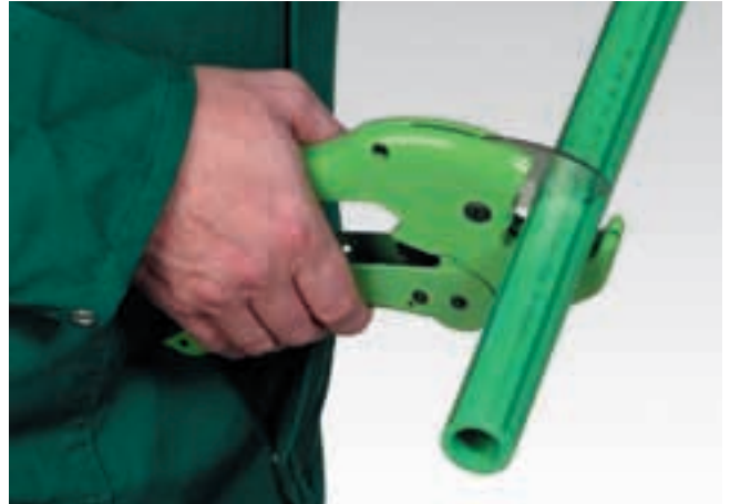
Cutting of the pipe
