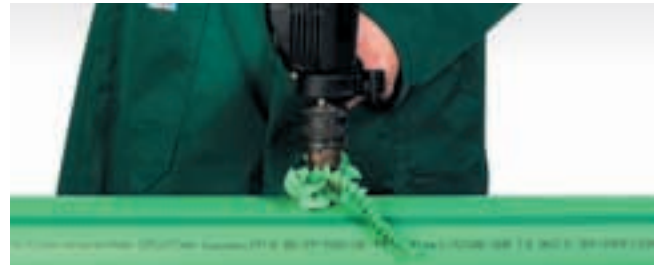
Drilling through the pipe wall
